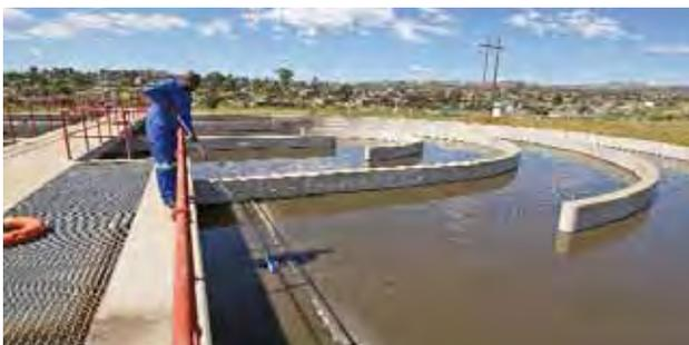
Agric College Activated Sludge Waste Water Treatment Plant
