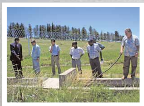
Handover of sewage treatment plant at TY by UNIK Construction and Engineering
