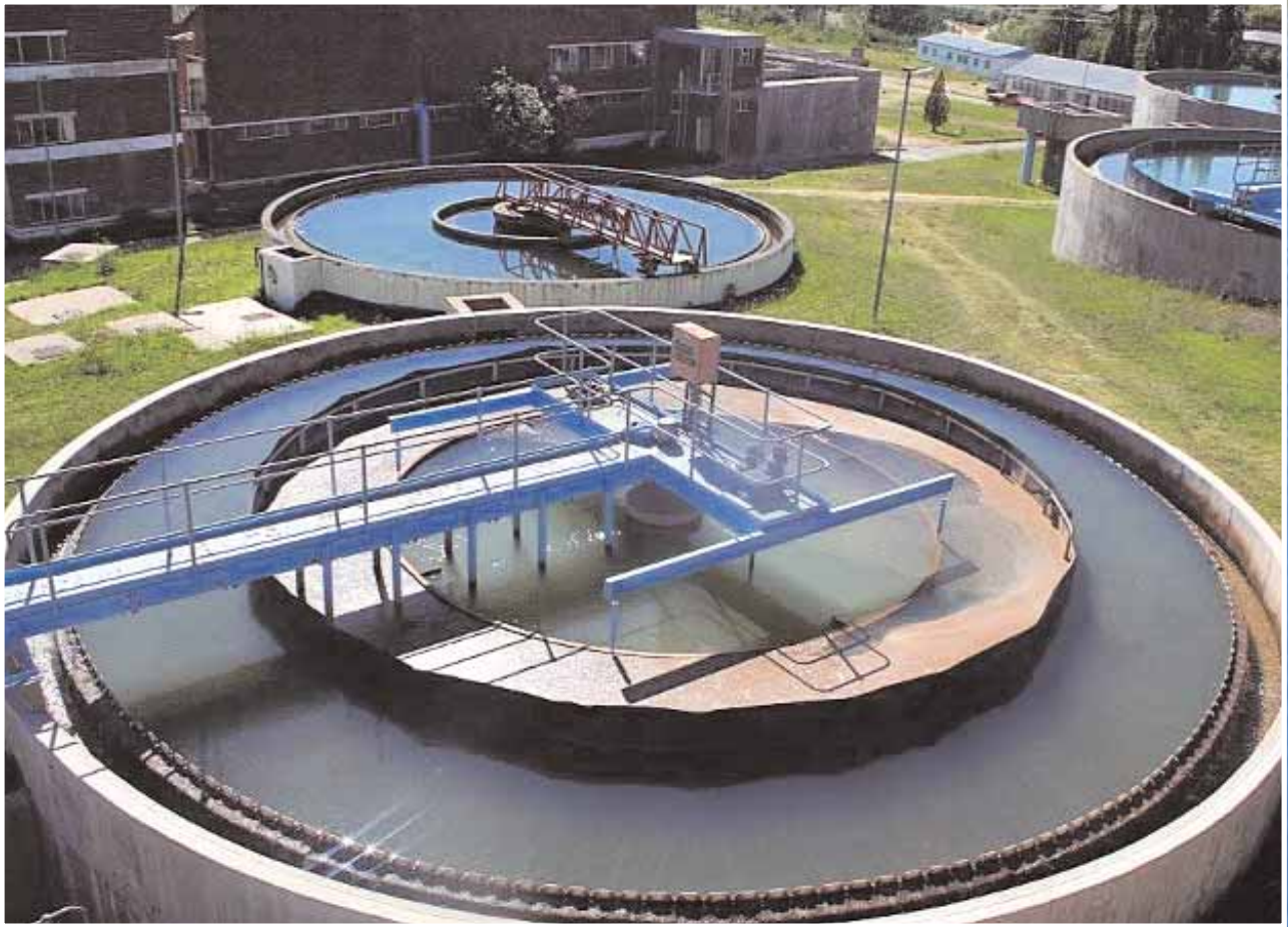
Maseru Water Treatment Plant
