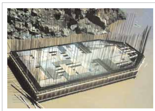
Construction of Maqalika Raw Water Pump Station
