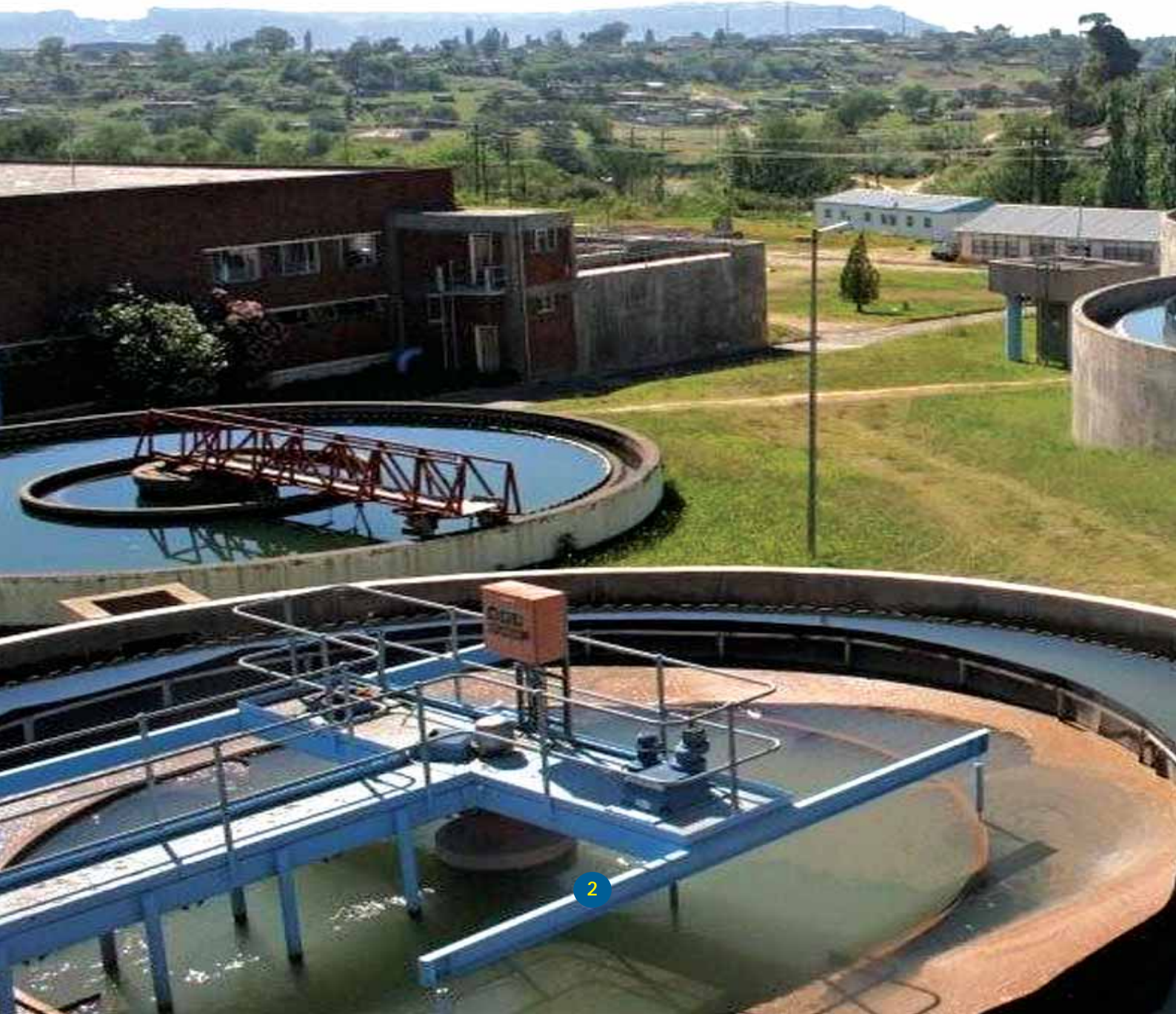
Maseru Water Treatment Plant
