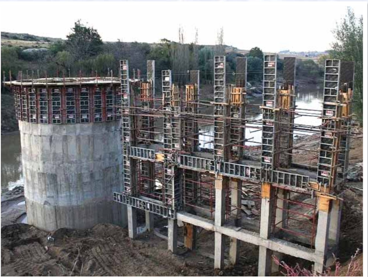
Water intake structure – Tikoe Thetsane Water Treatment Plant
