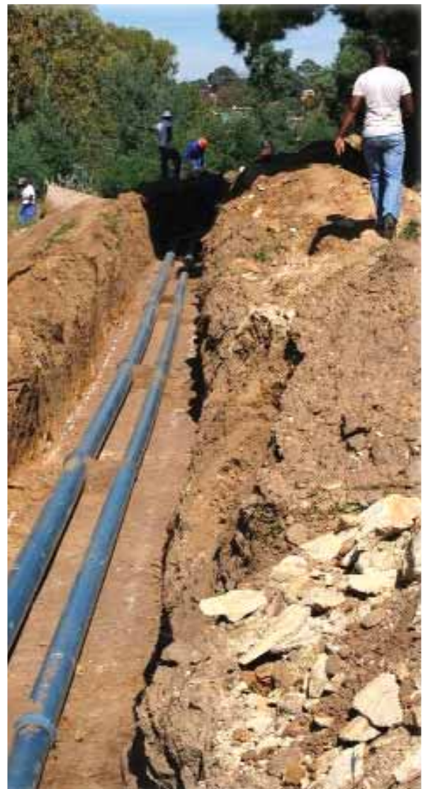
Pipe laying at TY town
