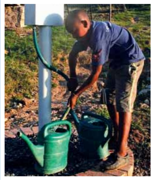
Communal prepaid standpipe at Mamenoaneng
