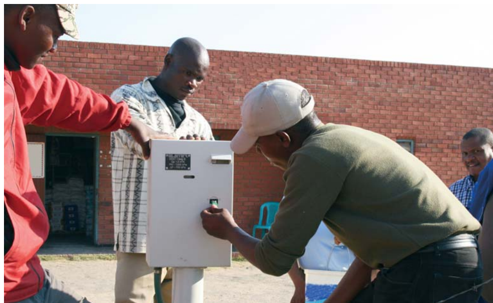
Communal Pre-paid metres.
