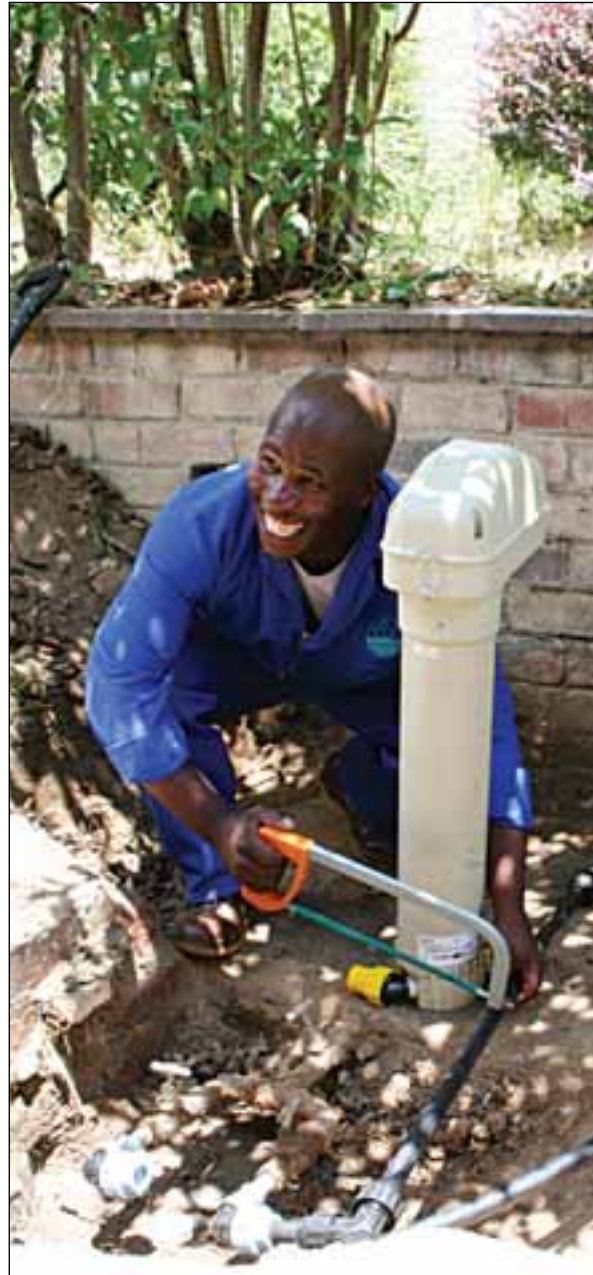
Installation of pre-paid meters in Maseru. 0
