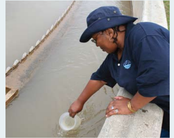
Ms. Engelina Motabo drawing a sample at the primary sedimentation tank for testing.
