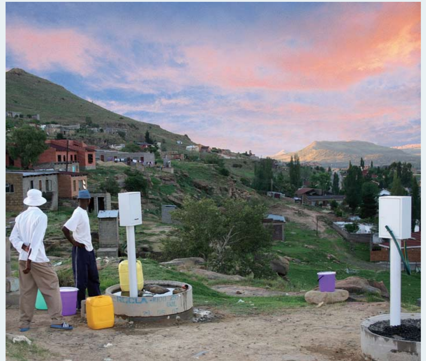
Two communal pre-paid standpipes at Ha Thetsane in Maseru City..
