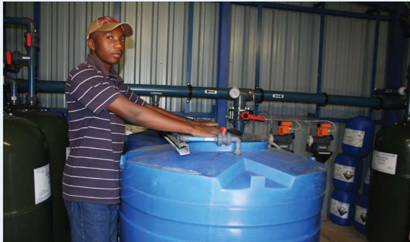
Mr. Pali Phafa at the mini water treatment plant Makhalaneng Roma.
