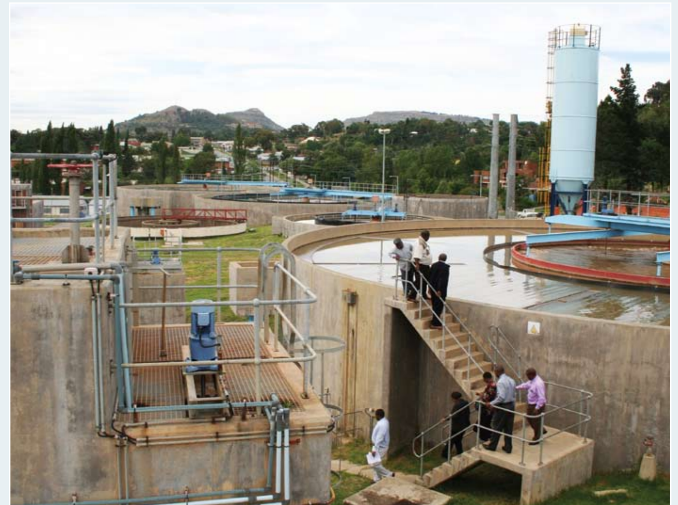
Maseru Water Supply purification plant.
