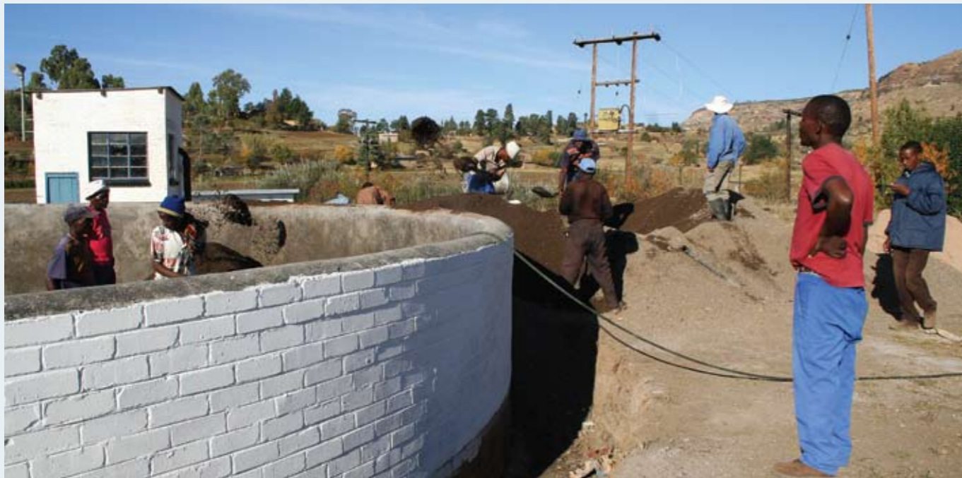
Rehabilitation of the filters at Butha Buthe Treatment Plant.
