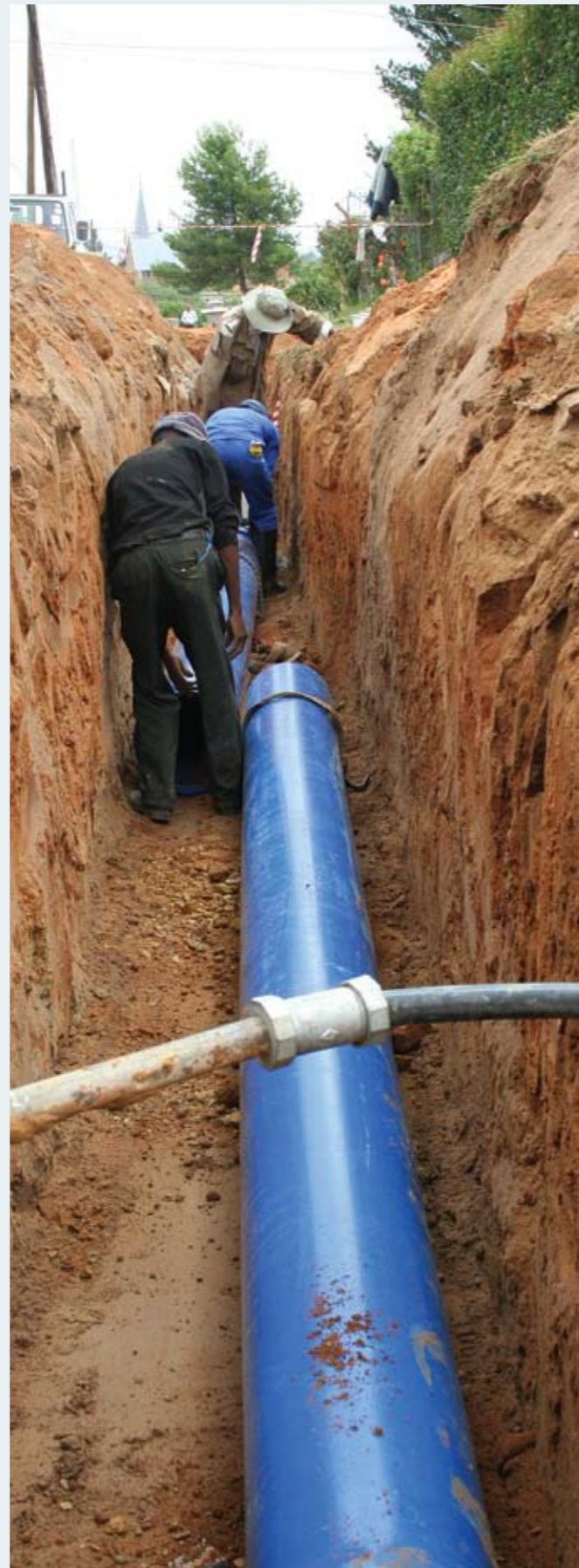
Pipe laying at Ha Tsoane under Maseru Peri-Urban Water Supply Project.
