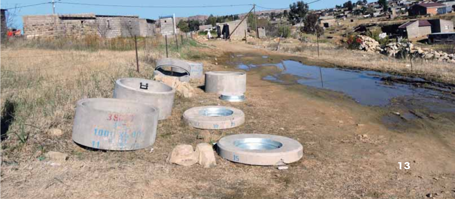
Concrete rings used in sewer connections
