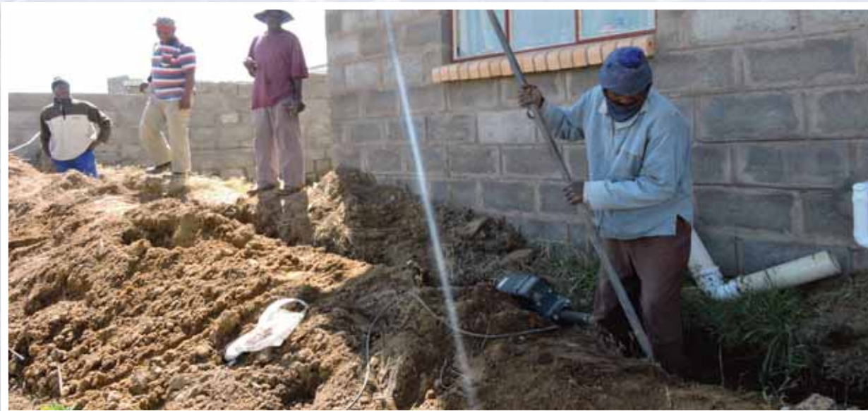
Sewer line connection construction works, ha Rankhala, Khubetsoana
